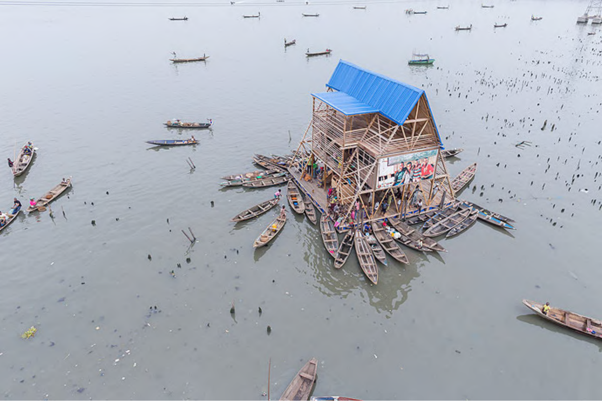
Makoko Floating School, Lagos Lagoon, Nigeria, designed by Kunle Adeyemi, NLE Architects
