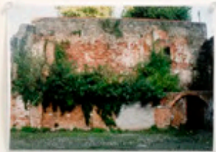
Brick building near the river, Clifton, 1st of March
